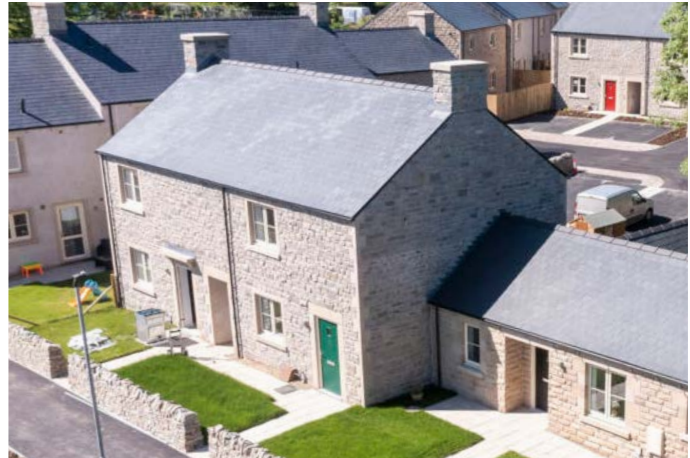
➤ Colonel Wright Close, Derbyshire. Platform Housing Group pride themselves in creating homes that integrate with their local setting, whether that be traditional or contemporary in architectural style.
